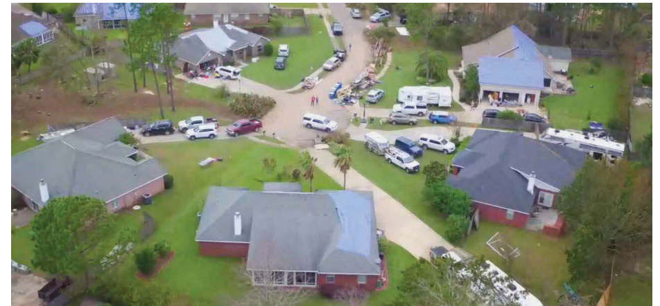
The fortified roof in Orange Beach, Ala. (bottom right, without a tarp) was not damaged by Hurricane Sally. Photo credit: Insurance Institute for Business and Home Safety
